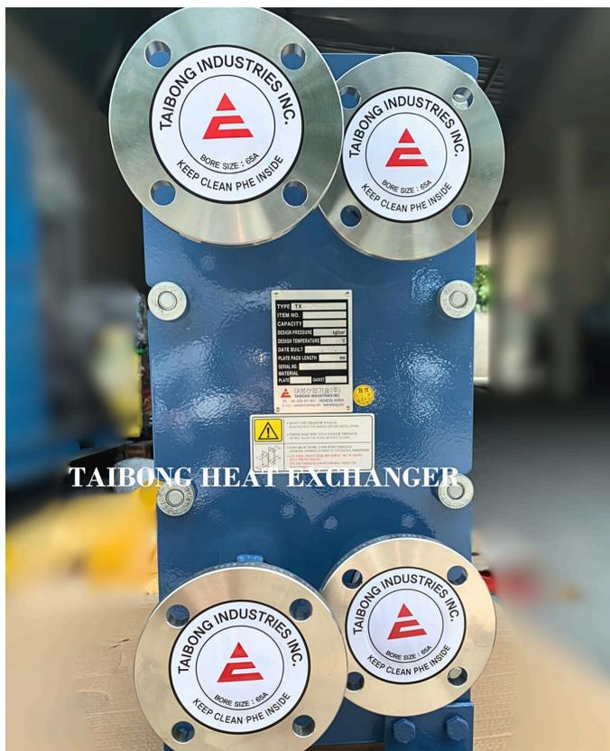
TX3GD plate can handle multiple responsibilities up to 40m<sup>3</sup>/h and heat capacity up to 400.000 kcal/h, in a single pass, meeting several application requirements.
